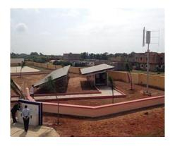
A self-sustaining water filtration system at the University of Kenitra in Morocco. Solar panels and a wind generator power the system that is visible under the right-most solar panels. From there, fresh drinking water is delivered to the taps in the foreground. (Credit: Firmus)
